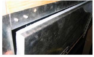
Ceiling type inlets should open at least 1 inch to insure a good air nozzle effect. Traditional sidewall inlets should open at least 2 inches (see photo on page 1).
