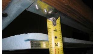
An inexpensive latch or nail to seal off unneeded air inlets is perhaps one of the best tools in setting up houses for good winter airflow. The number of inlets to be used must be matched to number of fans that will come on. During brooding and cold weather, a large number of the inlets must be closed off to assure good airflow.
